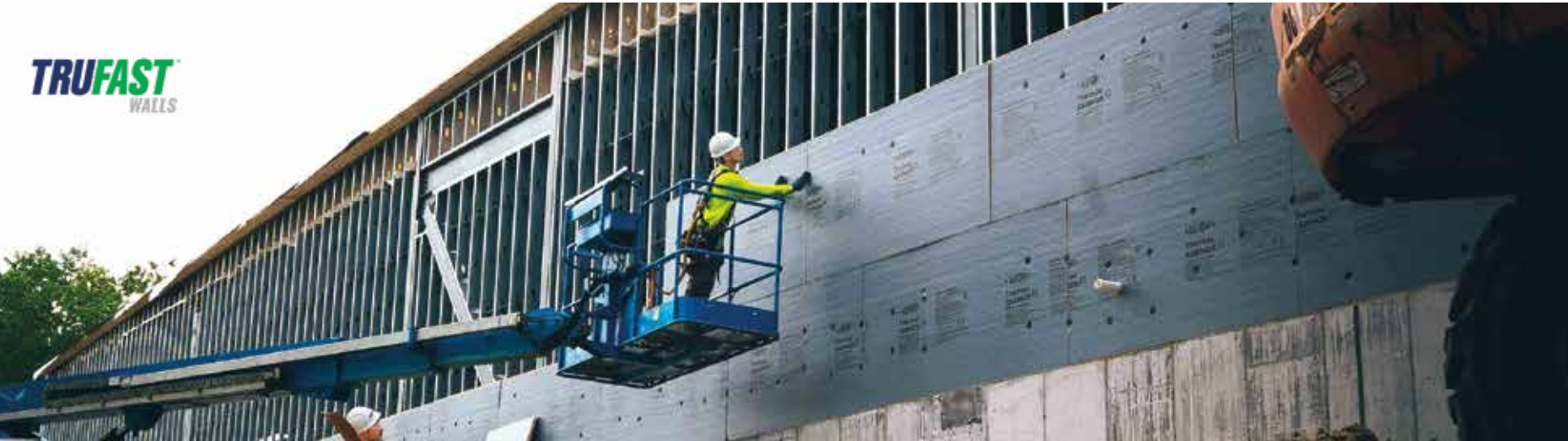
Installation of fastening systems from TRUFast Walls, a brand of ABC in the USA
