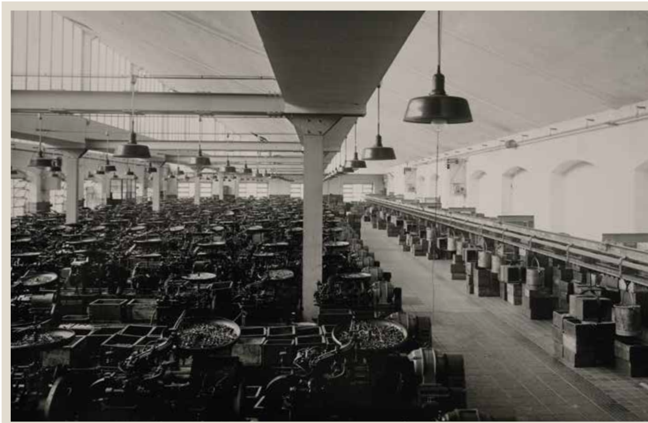
ABC turning shop in the 1930s: Production is electrified throughout, for lighting and machine drive alike. It provides jobs for numerous people.
